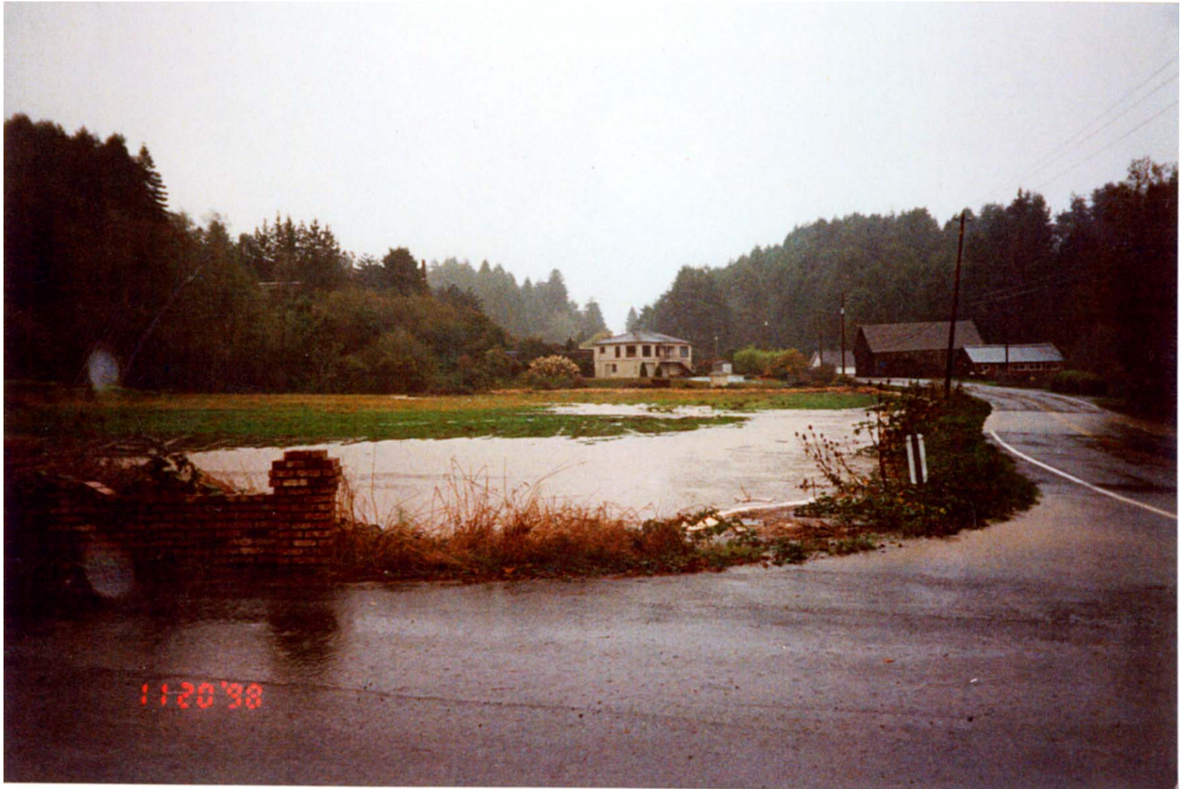
Figure 5. Floodwaters overtopping Old Arcata Road during the November 1998 flood. Photograph taken at the foot of Rocky Creek Road looking south. The main channel is in the distance; the secondary culvert entrance is in the foreground.
